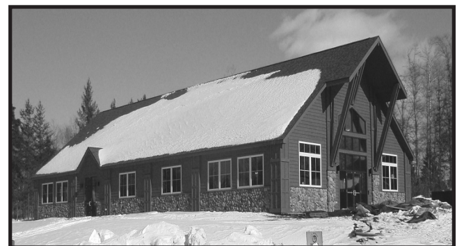
The new swimming pool at Whitebirch Estates.
