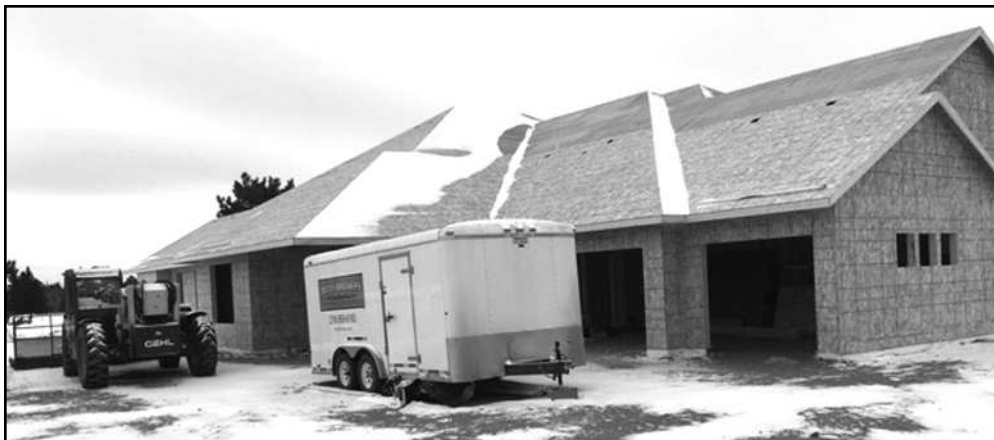
Construction continues on the Whitebirch Village townhomes.
