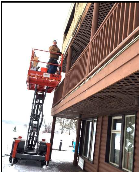
Workers replacing the railings along the walkways of Breezy Center.
